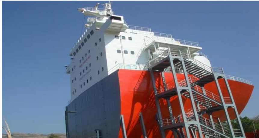
Ship-In-Campus – Outside View
