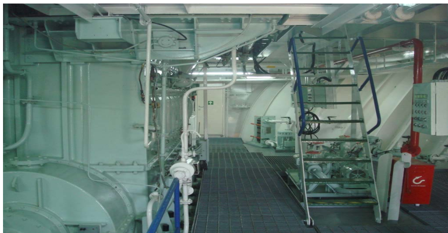
Ship-in-Campus – ER Bottom Deck
